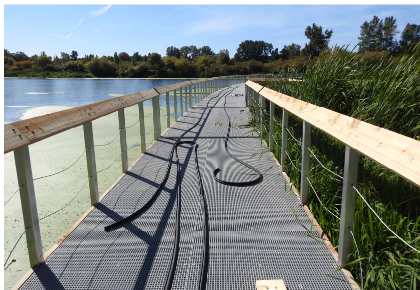
Figure 48. New aeration lines on boardwalk deck.
